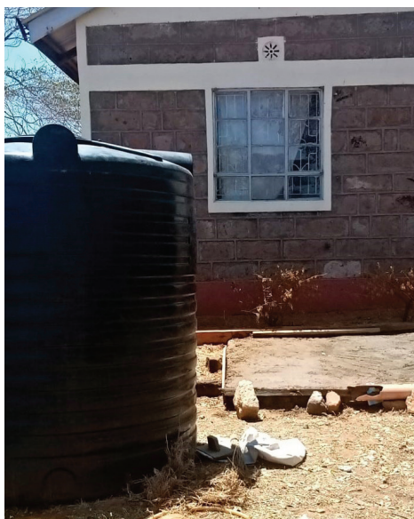
Installed water tank at Itunduimuni health centre
